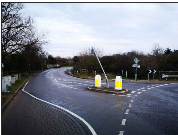
EXISTING ISLAND TO BE REMOVED
